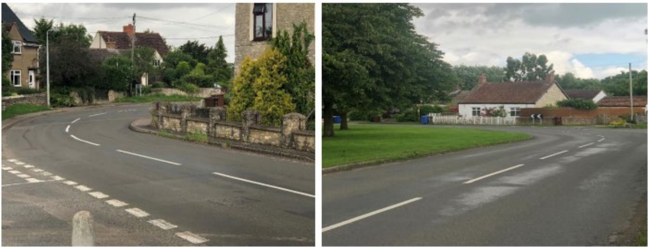
The two 90-degree bends with narrowing of road through the centre of Arccott Village
